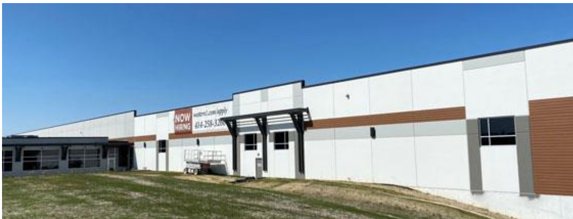
Western Building Products in Germantown, Wisc. featured 277 wall panels and 2, 200 square feet of hollow core.
